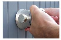
Step 5: Vacuum breaker is at the 9 o'clock position, and the spout is at 3 o'clock
